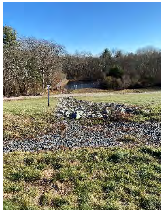
Photograph #12 Rip rap downchute to Basin 1 is in good condition.
