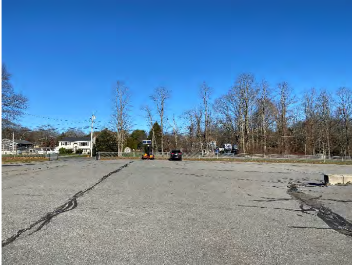
Photograph #5 Pavement cap in good condition and maintained.
