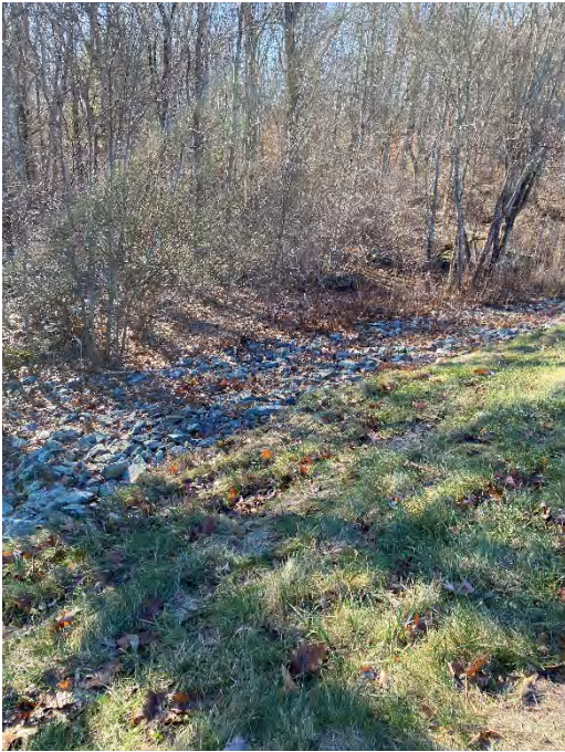
Photograph #21 Toe of slope rip rap protection.
