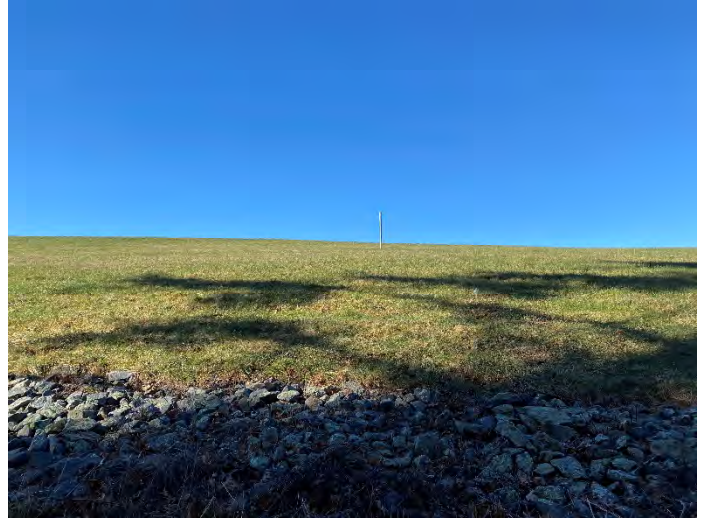
Photograph #22 Toe of slope rip rap protection.
