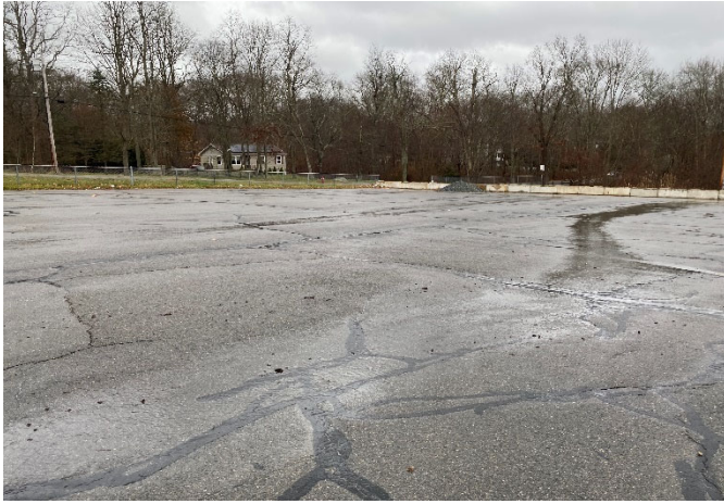
Photograph #5 Pavement cap in good condition and maintained.
