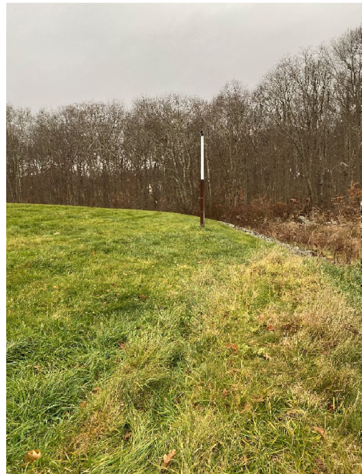
Photograph #24 Gas vents in good condition.
