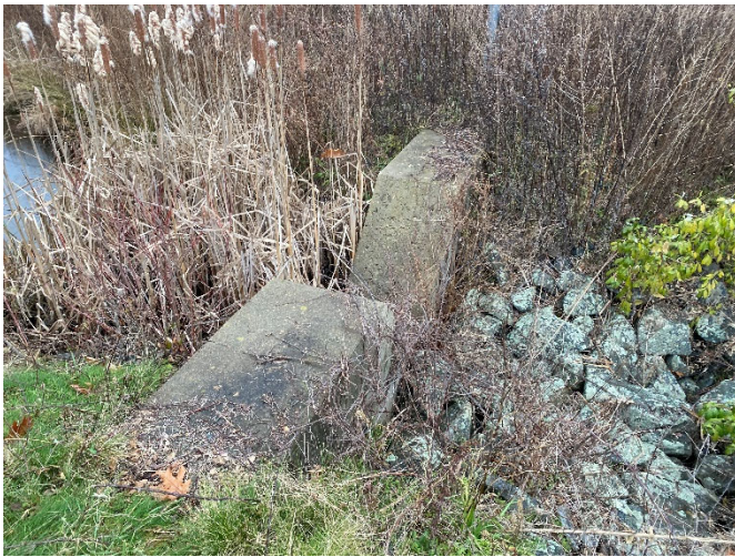
Photograph #7 V-notch weir at outlet from Basin 2.
