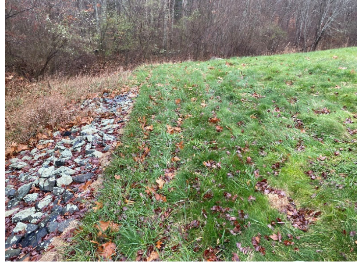
Photograph #22 Toe of slope rip rap protection.
