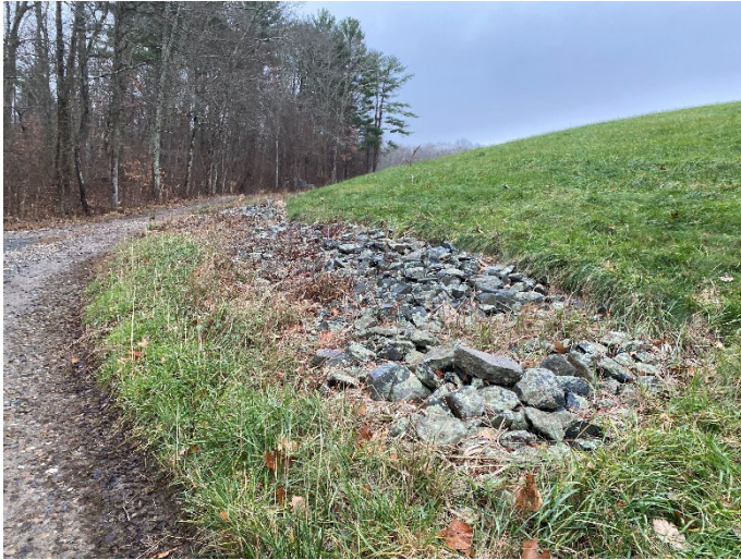
Photograph #21 Toe of slope rip rap protection.
