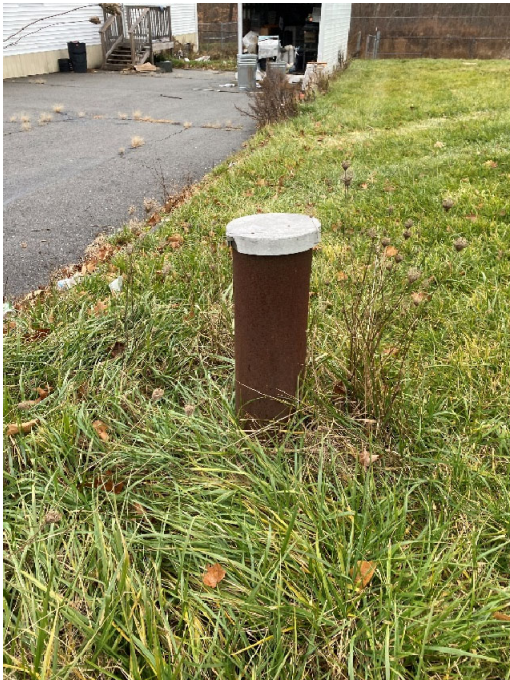
Photograph #25 Gas monitoring well GM-1.
