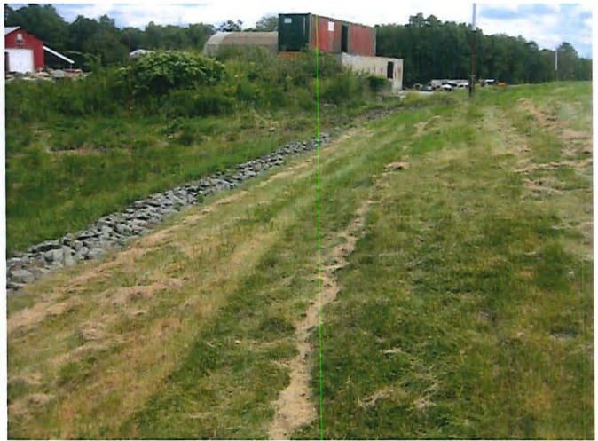
Photograph #22 Toe of slope rip rap protection.
