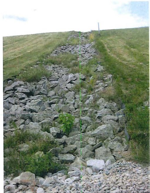
Photograph #12 Rip rap downchute to Basin 1 in good condition.
