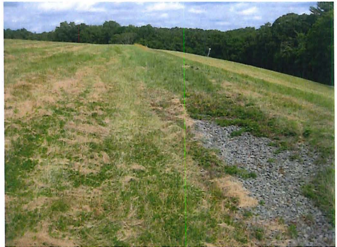
Photograph #14 Grass swales and rip rap section at top of downchute in good condition.
