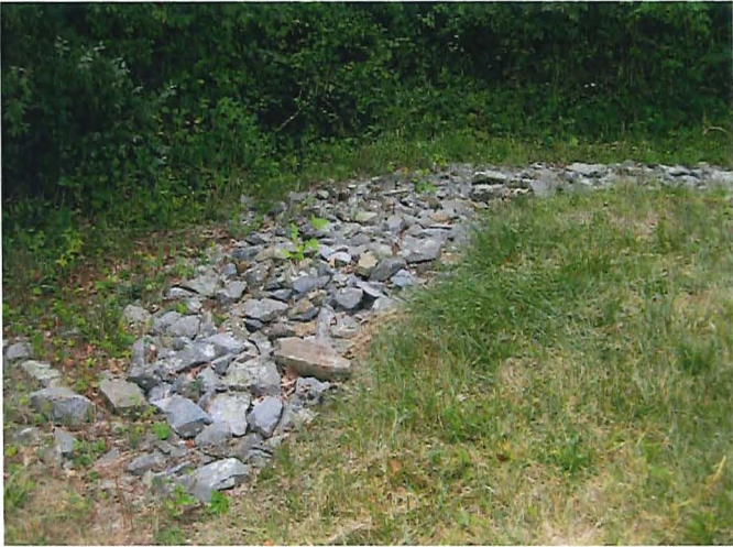
Photograph #21 Toe of slope rip rap protection.
