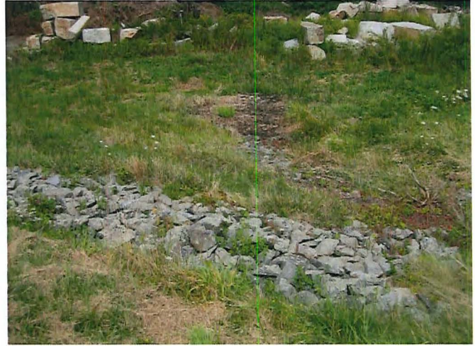
Photograph #10 Rip rap swale to small basin in northwest corner of the landfill.
