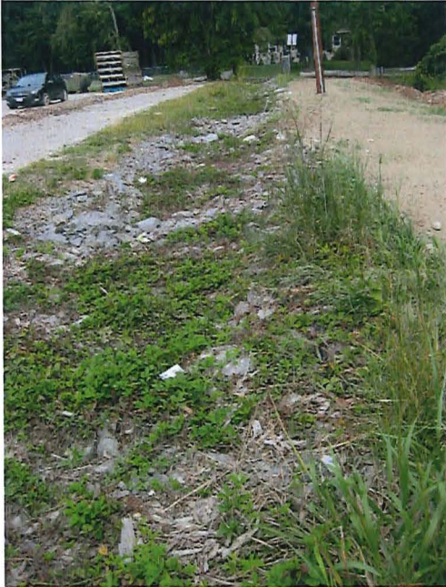
Photograph #13 Rip rap swale on east side of transfer station and edge of pavement cap in good condition.
