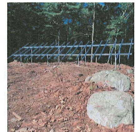
✓ Allows for mounting panels in four-, five- or six-high in landscape orientation and can be adapted to custom configurations
